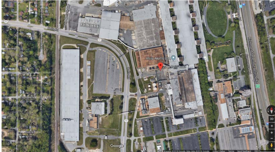
Figure 1. Location of the Manufacturing Facility
