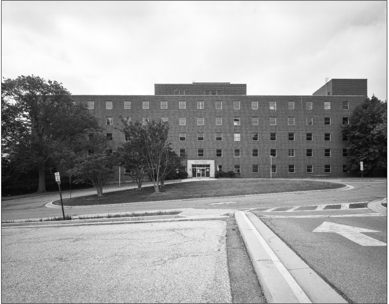
HABS photograph taken July 12, 2021, of Building 29, North Elevation. (Rob Tucher Photography)
