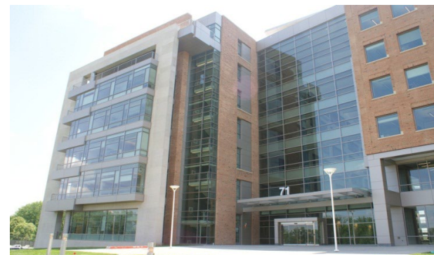
Building 71- Leadership and Administrative
