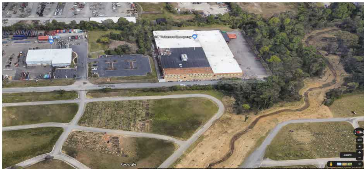
Figure 1. Location of the Manufacturing Facility 2
