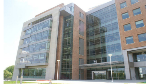
Building 71- Leadership and Administrative
