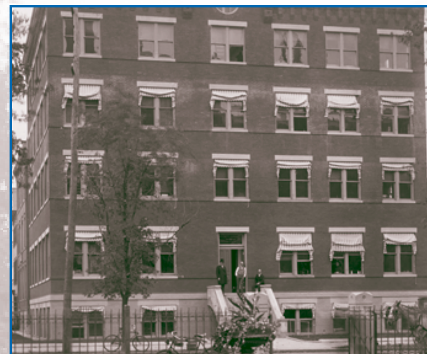
Dr. Harvey W. Wiley (in top hat), "Father of the Pure Food and Drugs Act," stands on the steps of the Bureau of Chemistry building in Washington D.C., as it was at the time of the 1906 Act.
