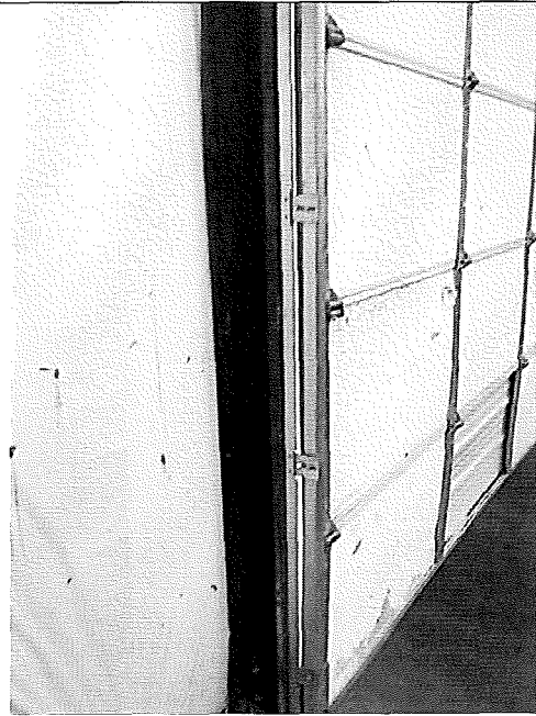
Obs. 1.c. Digital Photo 1568 – A gap approximately 1/2 inch wide by 10 feet high, was observed along the north side of the dock door.
